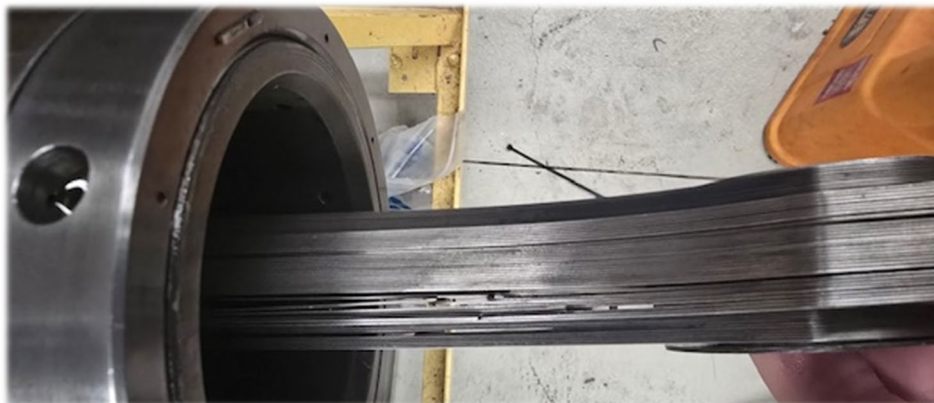
Figure 1. Subject failed segments of Main Rotor Tension Torsion Strap
