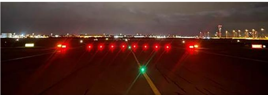
Figure 9. Holding point stop-bar lights
