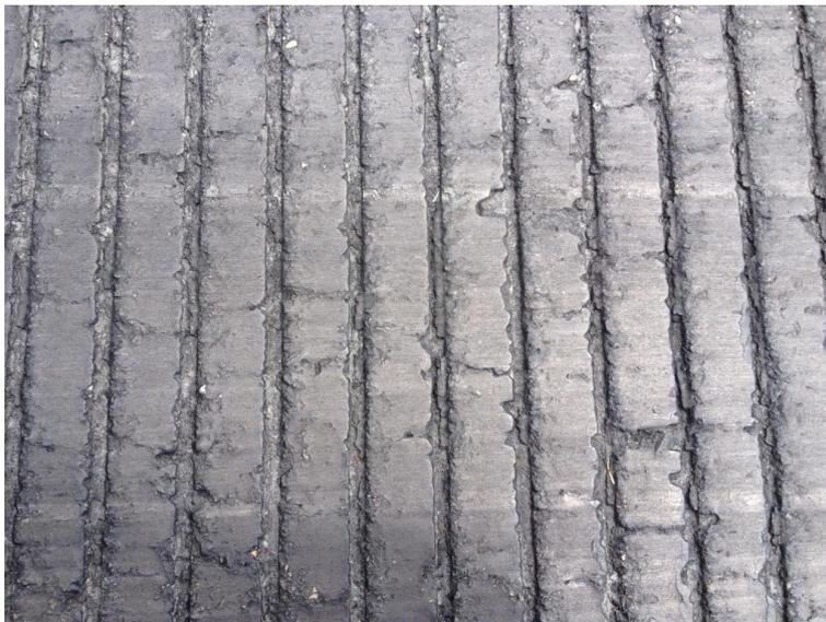
**Figure 17. Example rubber contamination of a grooved runway.**
