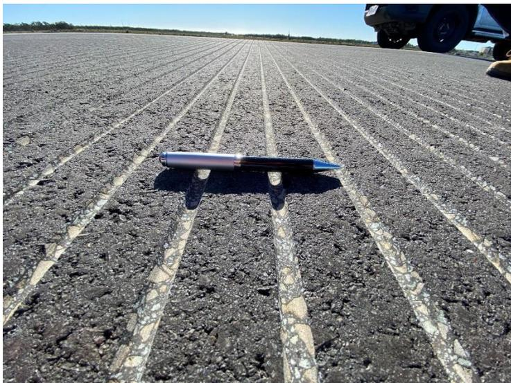
**Figure 11. Typical trapezoidal grooves in DGA surface.**
