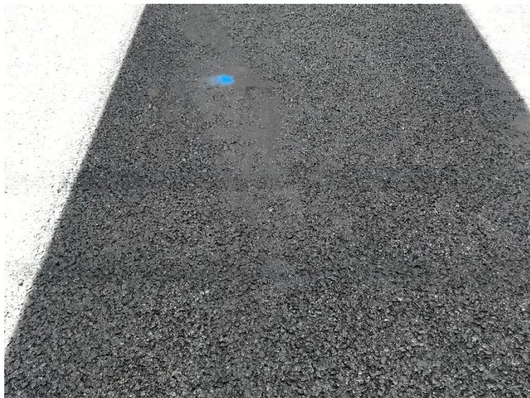
**Figure 14. Example of isolated asphalt bleeding in SMA.**
