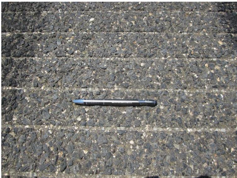
**Figure 19. Example of severely eroded grooved surface.**
