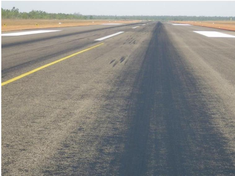
**Figure 13. Example of wheel path flushing of a sprayed seal.**
