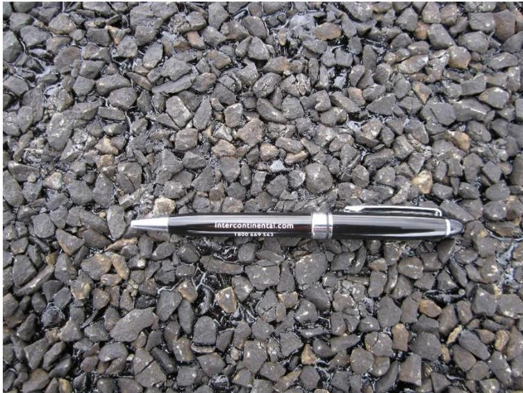
**Figure 2. Typical sprayed seal runway surface.**
