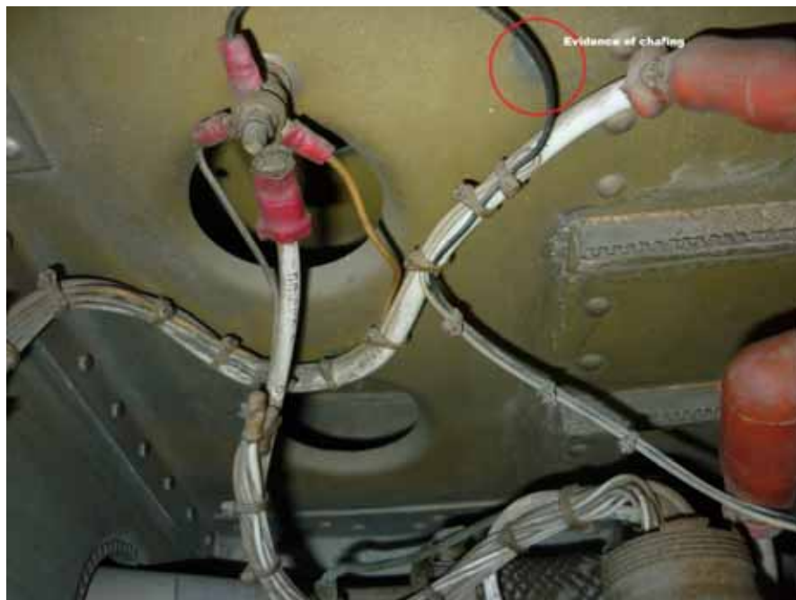
Figure 5 – Wire routing for starboard inverter.
